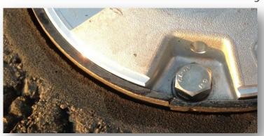
Make sure the specified tightening torque is applied
